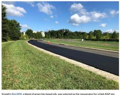
demonstration project in Ashburn, Virginia. ReLIXER softens and restores the functional properties of the aged binder in RAP, aids workability and compactability of the asphalt mix, delivers the required roadway performance and durability, and reduces the need for virgin binder.
