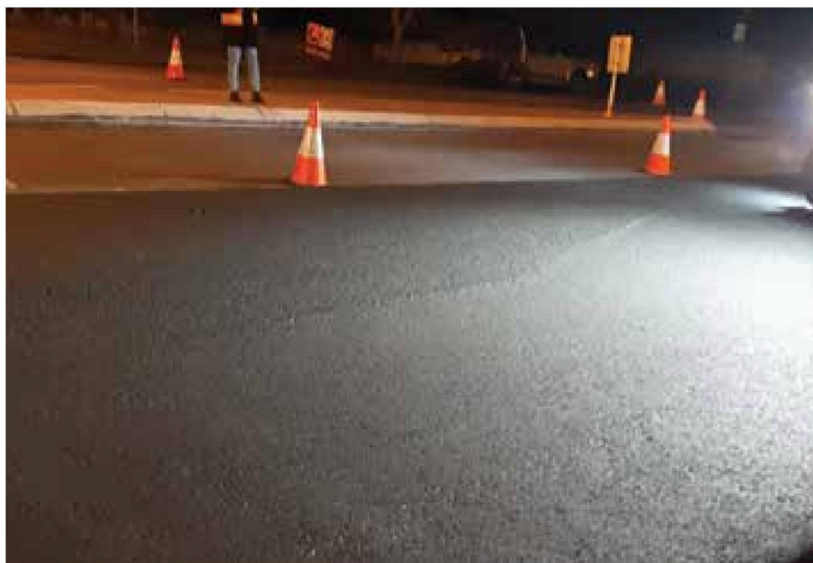
High-RAP mixes with ReLIXER on roadway in Brisbane City, Queensland, Australia
