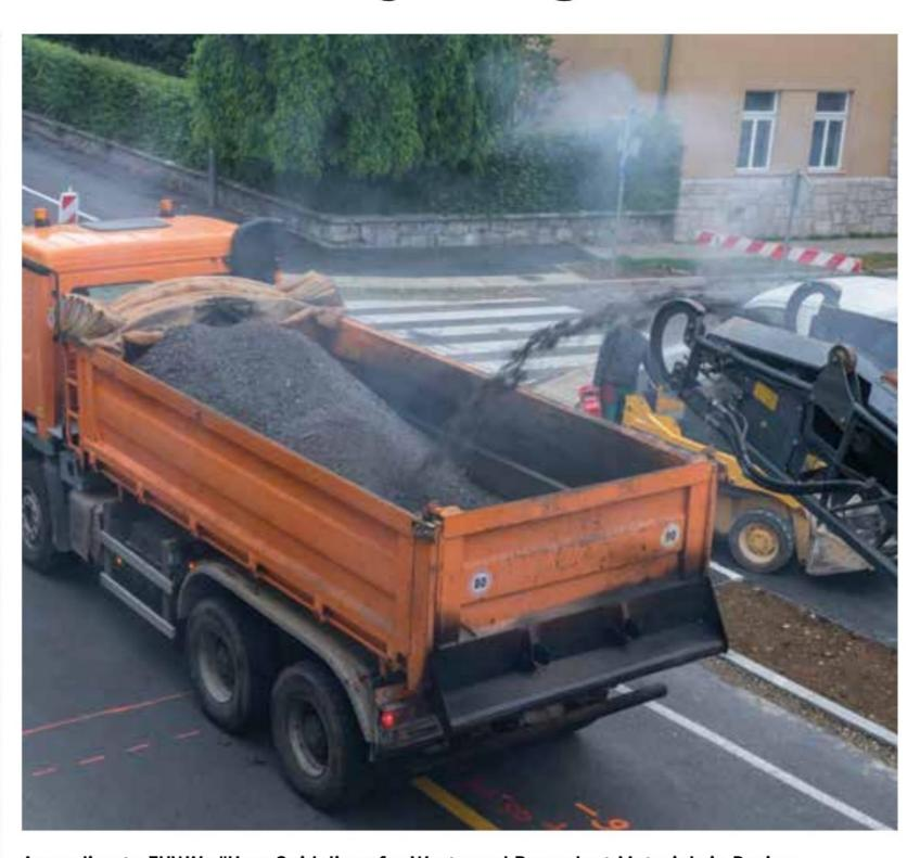
According to FHWA's "User Guidelines for Waste and Byproduct Materials in Paving Construction," from FHWA, roadway milling produces over 45 million tons of RAP in the U.S. annually. *Photo courtesy of Sripath Technologies*
