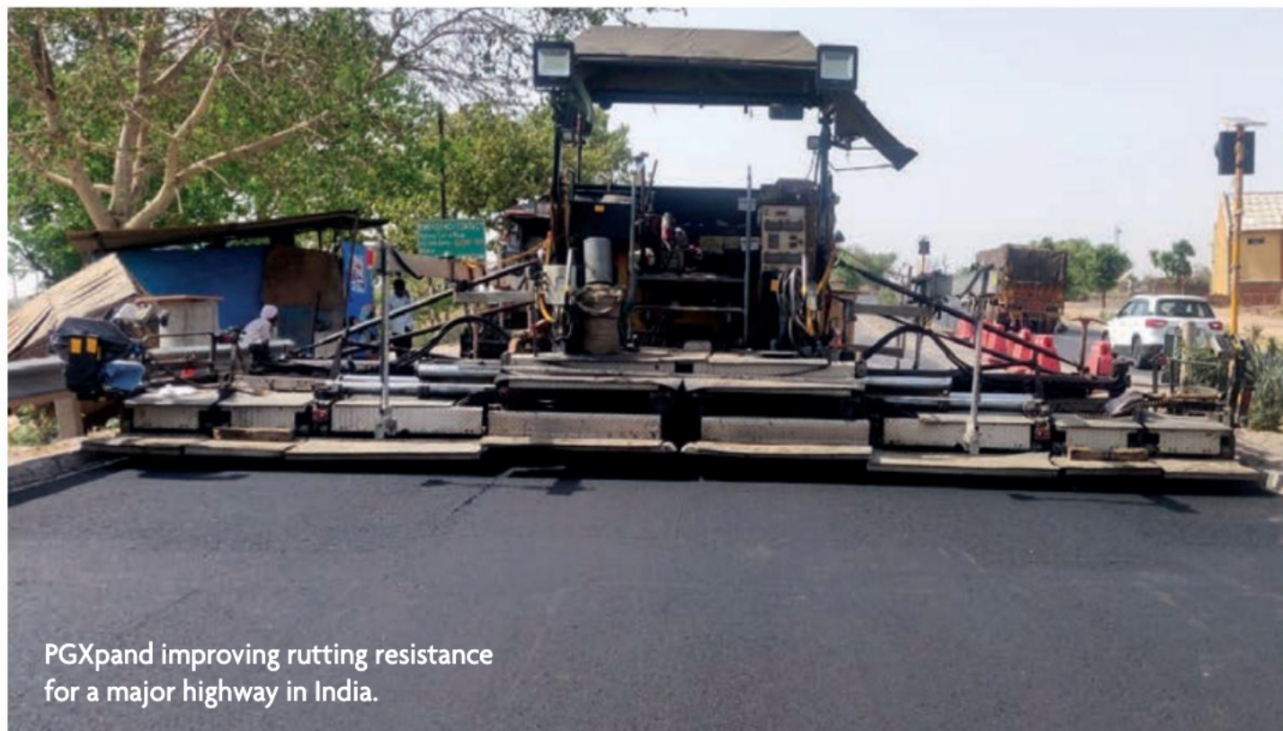
A polymer modified bitumen and PGXpand mix being paved on a roadway.
