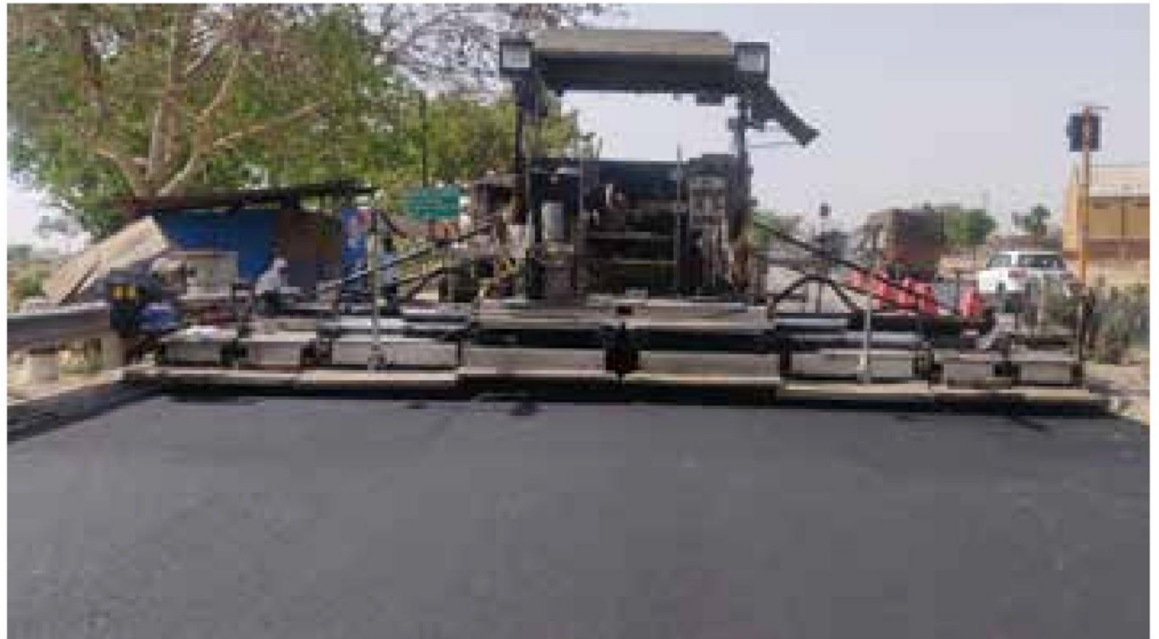
Sripath PGXpand® modified bitumen is placed on a field trial to improve rutting performance of a major highway in India.
