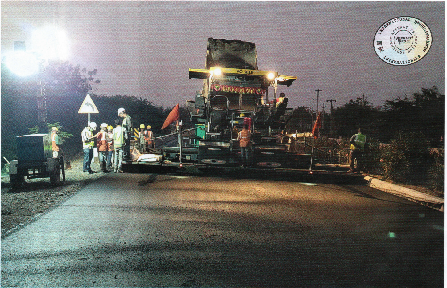
This successful paving trial used Sripath Technologies' PGXpand to lay down a wear layer surface in Andhra Pradesh, India. Photos courtesy of Sripath Technologies
